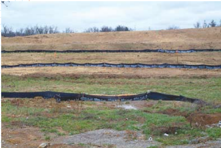
Use multiple silt fences at proper spacing (see table) to protect long, unvegetated slopes. Fences provide only temporary protection and can be removed when the area is seeded and mulched.
